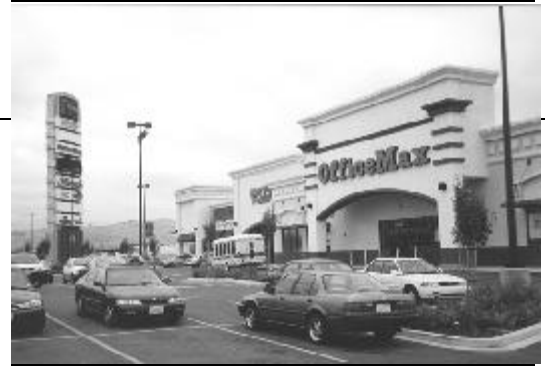
Office Max development in Union Landing with freeway pylon sign in background
