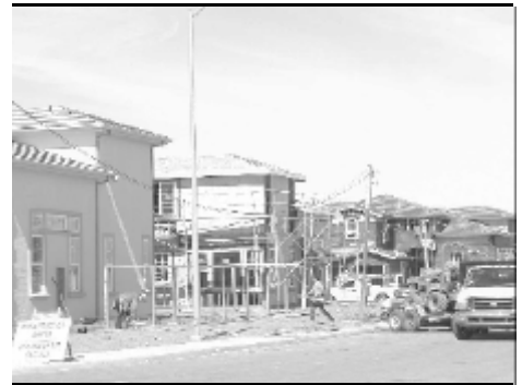
New home construction
