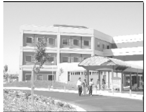
Kaiser Permanente campus expansion of medical office building
