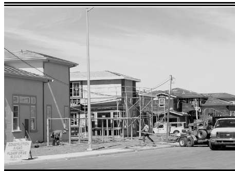
New residential construction
